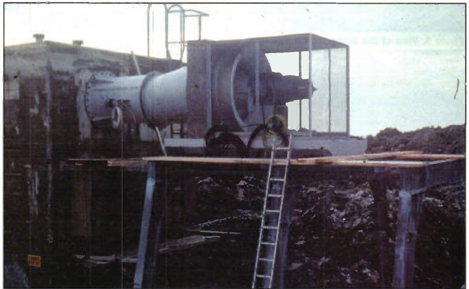
Photo 1. Original Wells turbine facility during construction on Islay (Courtesy ETSU)
