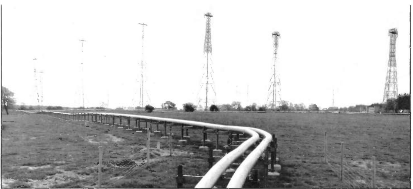
The HF transmitters (also known as 'senders') at Rampisham, in Dorset.
