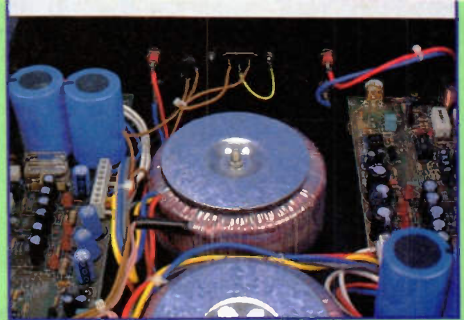
Rear panel wiring.
