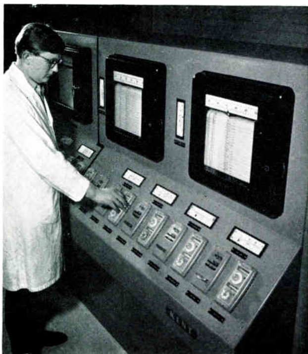
This shows the plant operator making adjustments to a 'Transdata' controller on the instrument console
