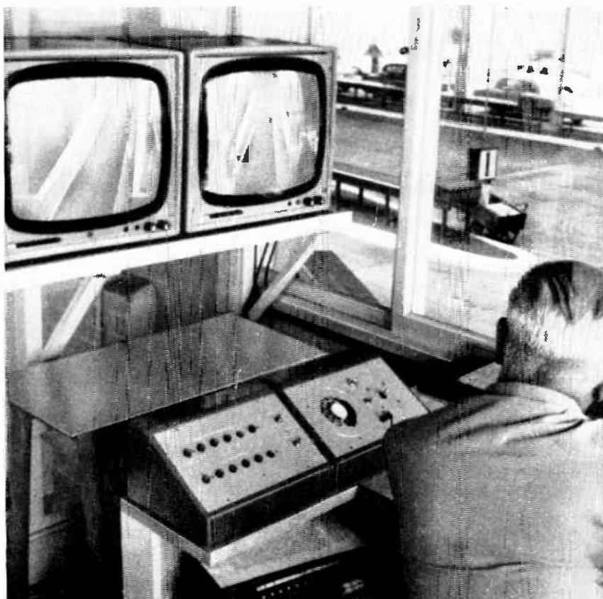
The picture on the left shows one of the cameras overlooking the entrance to the car-ferry terminal. Shown on the right is the control room where pictures from cameras installed by the ferry berths can be seen on the monitor screens. A telephone dialling system (shown below screens) enables the cameras to be controlled remotely so that focus, rotation and tilt can be adjusted
