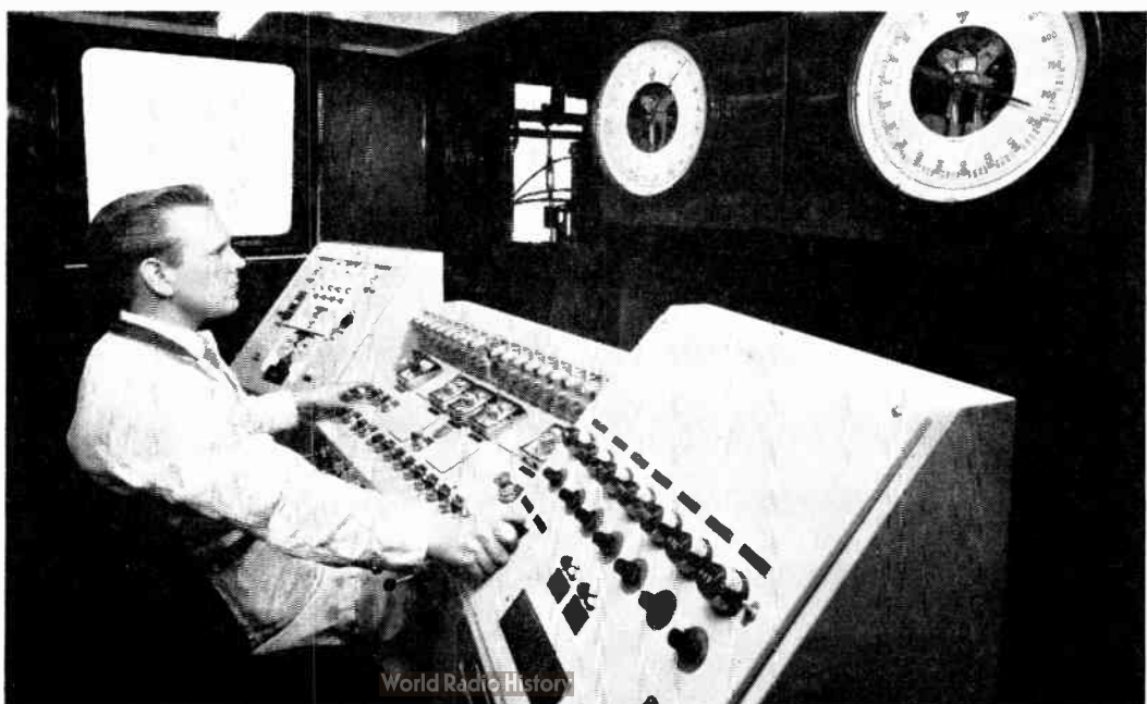
The control console
