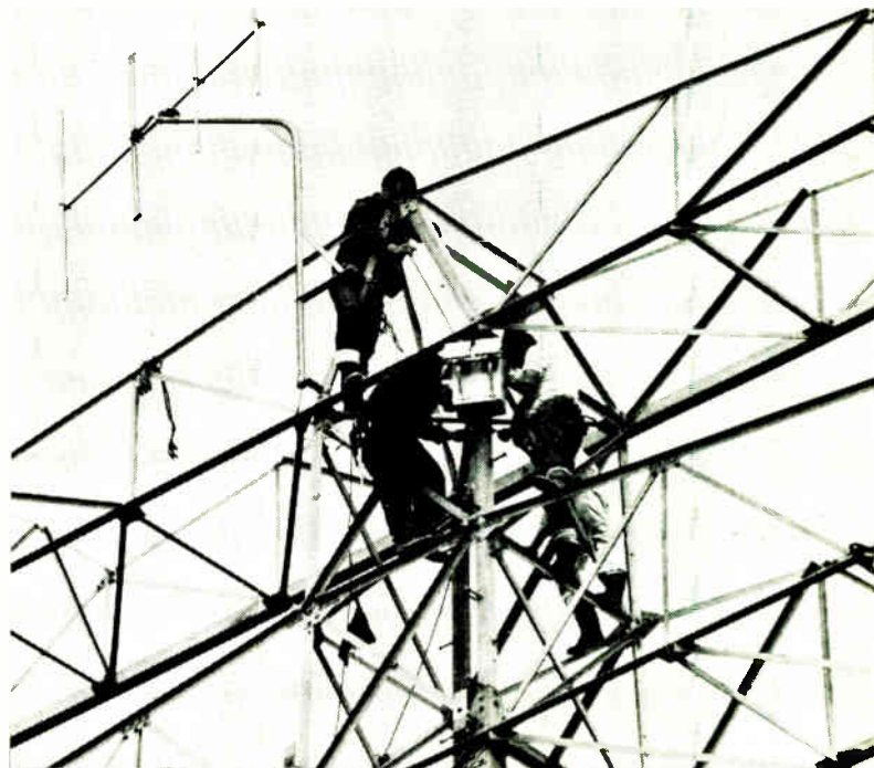
This shows one of the solar-powered transmitters being mounted on a high voltage transmission-line tower
