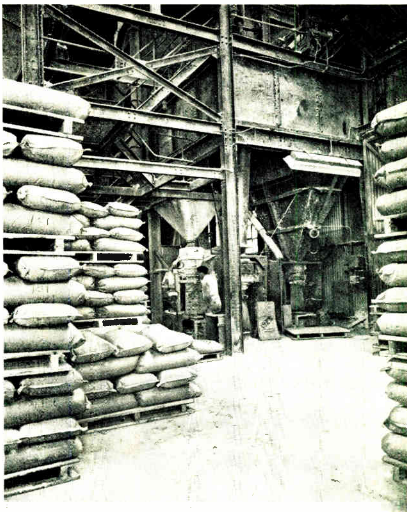
Bagging station of mill producing silica flour from dried sand
