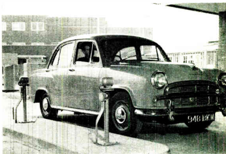
The projectors and receivers installed at the entrance to the building can be clearly seen in this picture
