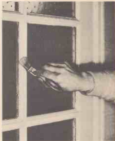
Cutting in round the windows—the most difficult job!
