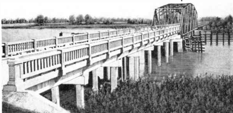
The Savannah River Bridge is the main bridge on the Atlantic Coastal Highway connecting Georgia with South Carolina, just on the outskirts of Savannah.
