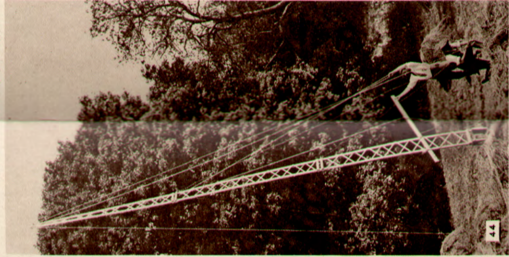
43 The complete lattice mast is assembled and bolted together on the ground, and then erected by pulling on the guy ropes as seen in the photograph
