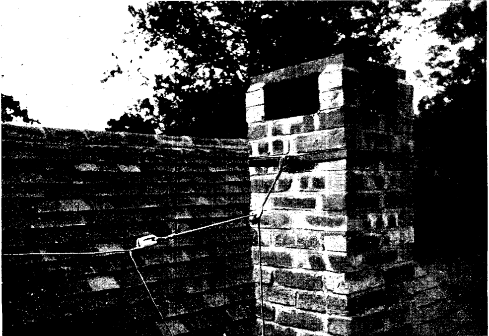
Fig. 29. How a galvanized iron strap should be fixed round a chimney to take the aerial wire. This method is adopted to avoid wall hooks, which have to be driven into the mortar
