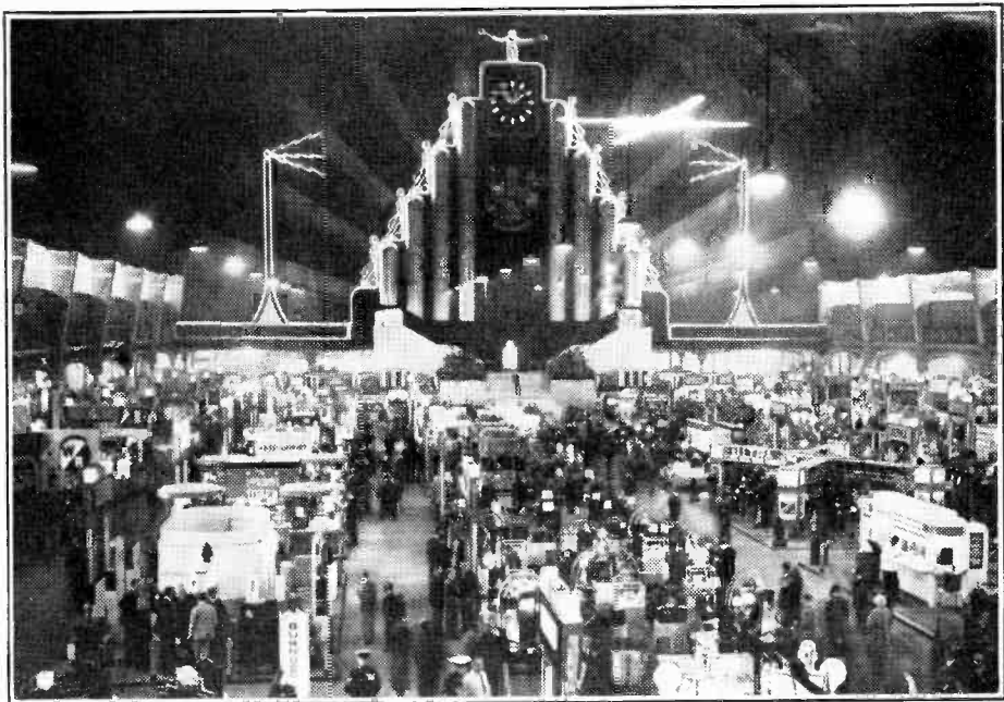
OLYMPIA RADIO SHOW, 1934. —A general view of the Main Hall, Olympia, on the opening day of the Radio Show. An illustrated report on matters of technical interest exhibited will appear in our next issue.
