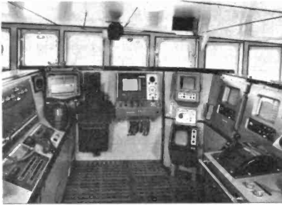
The "fishing cockpit" at the starboard side of a modern trawler's bridge. From the left the units are: crew call controls, Decca navigator, a radar set, four recording and one cathode ray tube echosounders, and propeller pitch adjustment for fine speed control.
