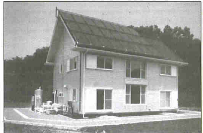
Figure 7: A Japanese house fitted with 1.8 kW of peak solar capacity by BP Solar as part of the New Sunshine Project. (Courtesy BP Solar Ltd.)
