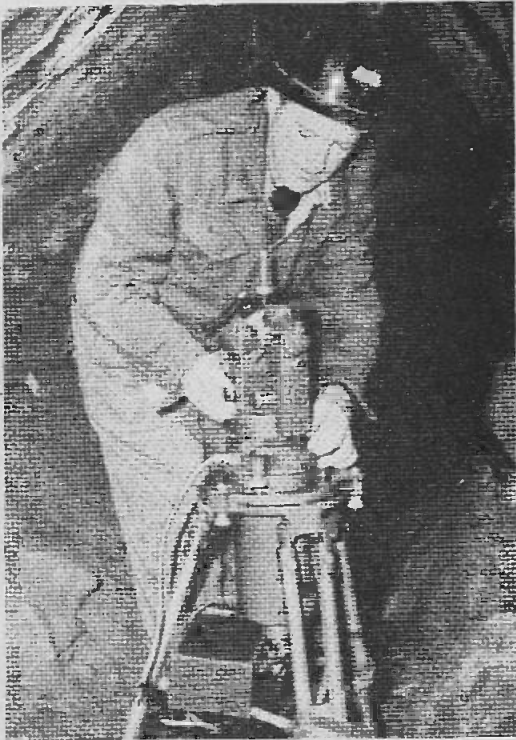
Fig. 12. A surveyor measuring underground with a gyro-assisted theodolite.
