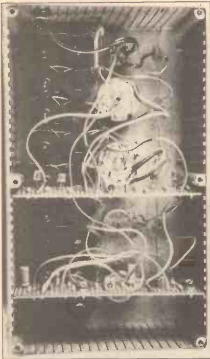
Interior view with veroboards in position.
