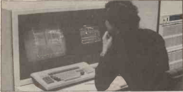
Colour graphics system allows analysis of complex integrated circuit chip layout.
