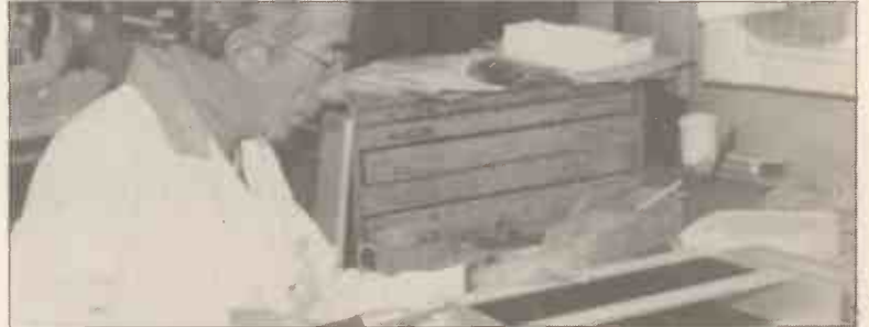
A 19" card frame being assembled.
