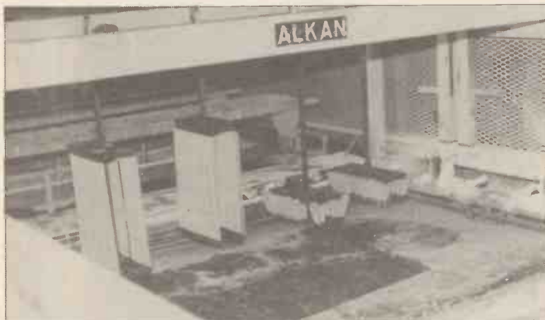
Chemical preparation (anodising) of the aluminium to give its high quality finish.
