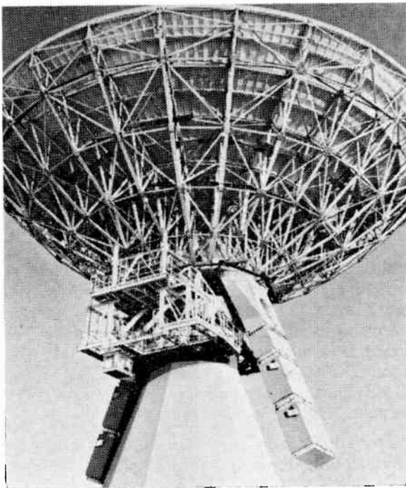
Fig. 6. Close-up detail of the dish backing structure.
