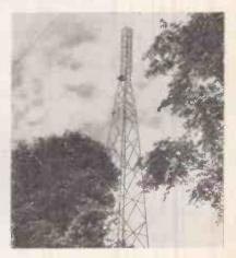
The Marconi mast and aerial, erection of which is completed, at the Croydon I.T.A. TV transmitting site. The aerial is a twin 4-stack Brnd III vertically polarised array. Meanwhile installation of the sound transmitter is complete, and the installation of the vision transmitter is going according to exhaust according to schedule.
