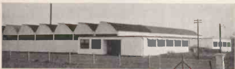
Aerfalle's new factory, situated at West End, Congleton, Cheshire, has been bought specially for the manufacture of television aerial equipment, converters, and electronic components.
