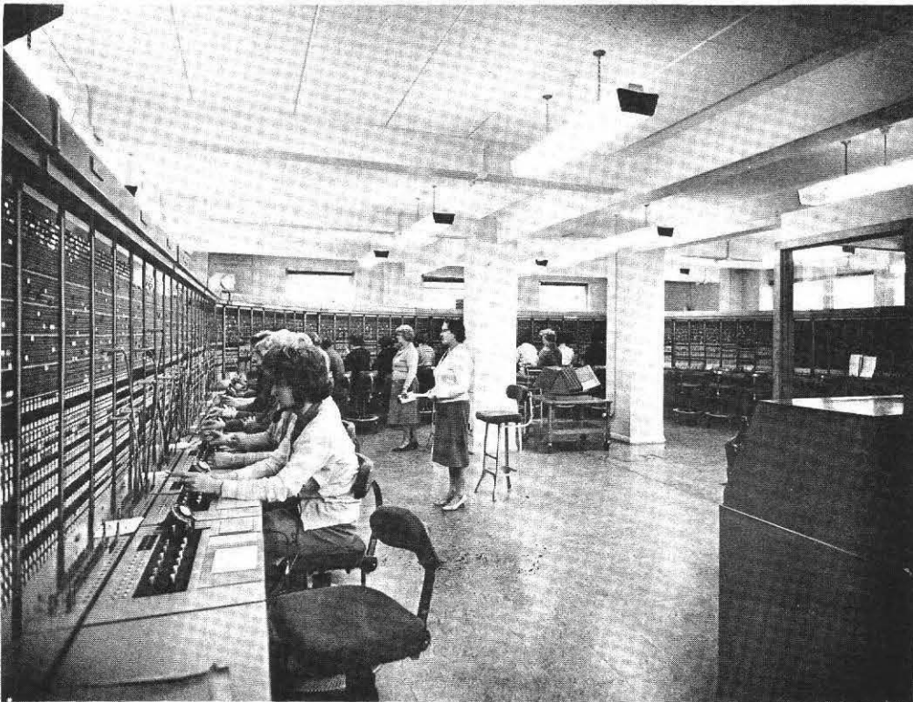
Plate II— Manual Board of Private Automatic Branch Exchange (PABX), Broadcasting House, London.
