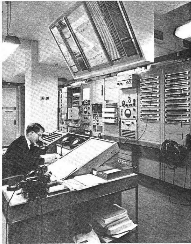
RIGHT, Plate III— Communications Room at Broadcasting House, London, showing Control Desk, testing apparatus, and main circuit interception equipment.
