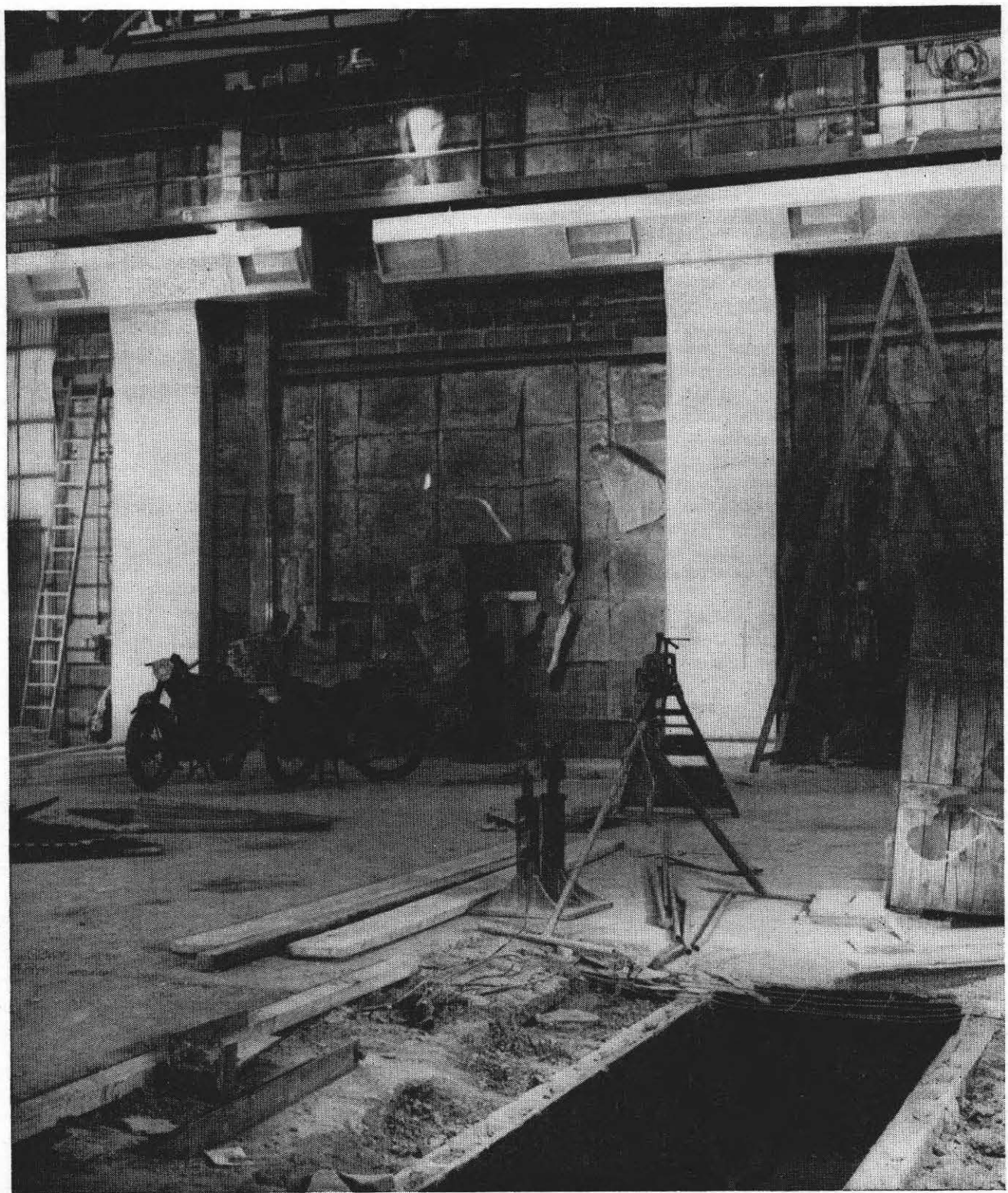
Plate A — Progress photograph showing underground vent ducts and vertical metal risers in Studio 1
