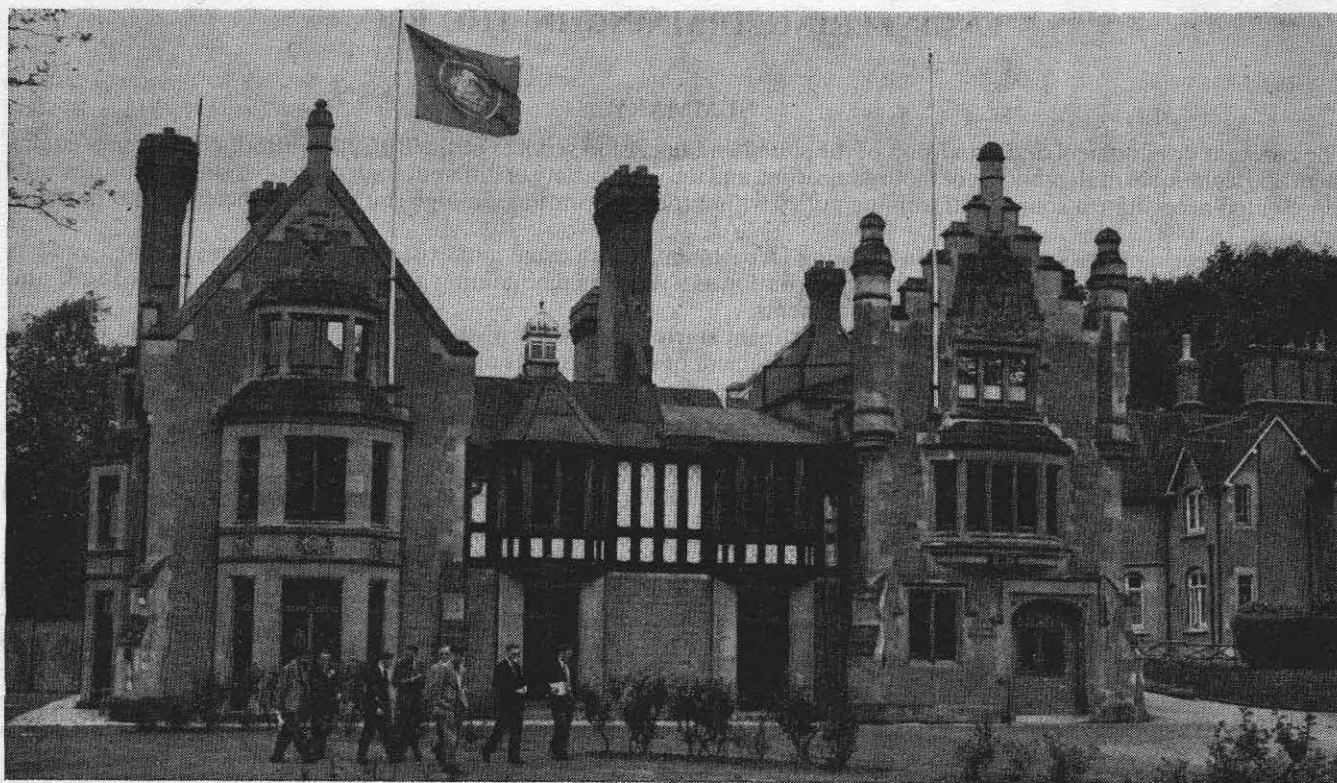
Fig. 1 — The main building, Wood Norton Hall
