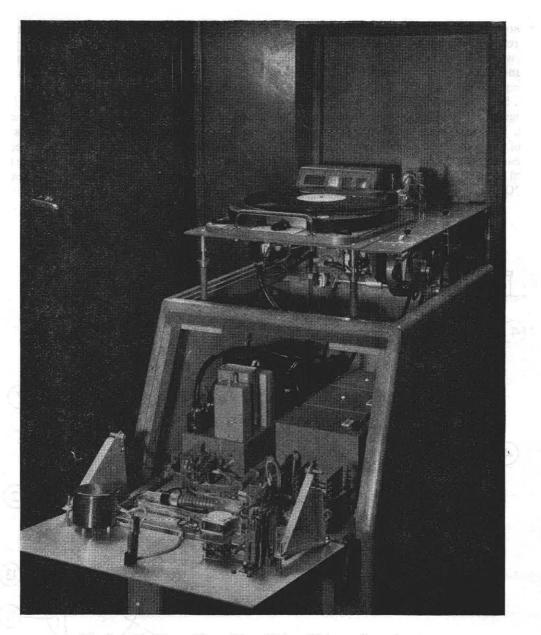
Fig. 3 — The Turntable and Tray Units withdrawn for maintenance
