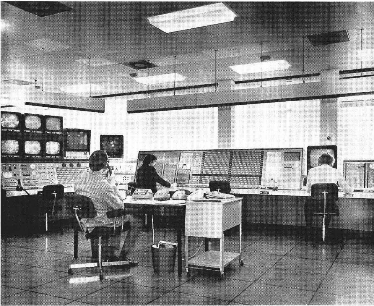
Fig. 2 Main control desk in the Communications Centre. The left-hand section beneath the monitor stack deals with vision (and television sound) switching and routing, pulse chain control, and vision measurement. The section from centre to right is concerned with sound (Radio) switching and routing, EMX, and control line routing. The main part of this section is the S.B. switcher (centre right). Beneath the left-hand colour monitor is the married switcher for television (vision and sound) routing
