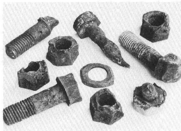
Fig. 7 The fate of steel nuts and bolts unprotected by galvanising and exposed for 40 years.
