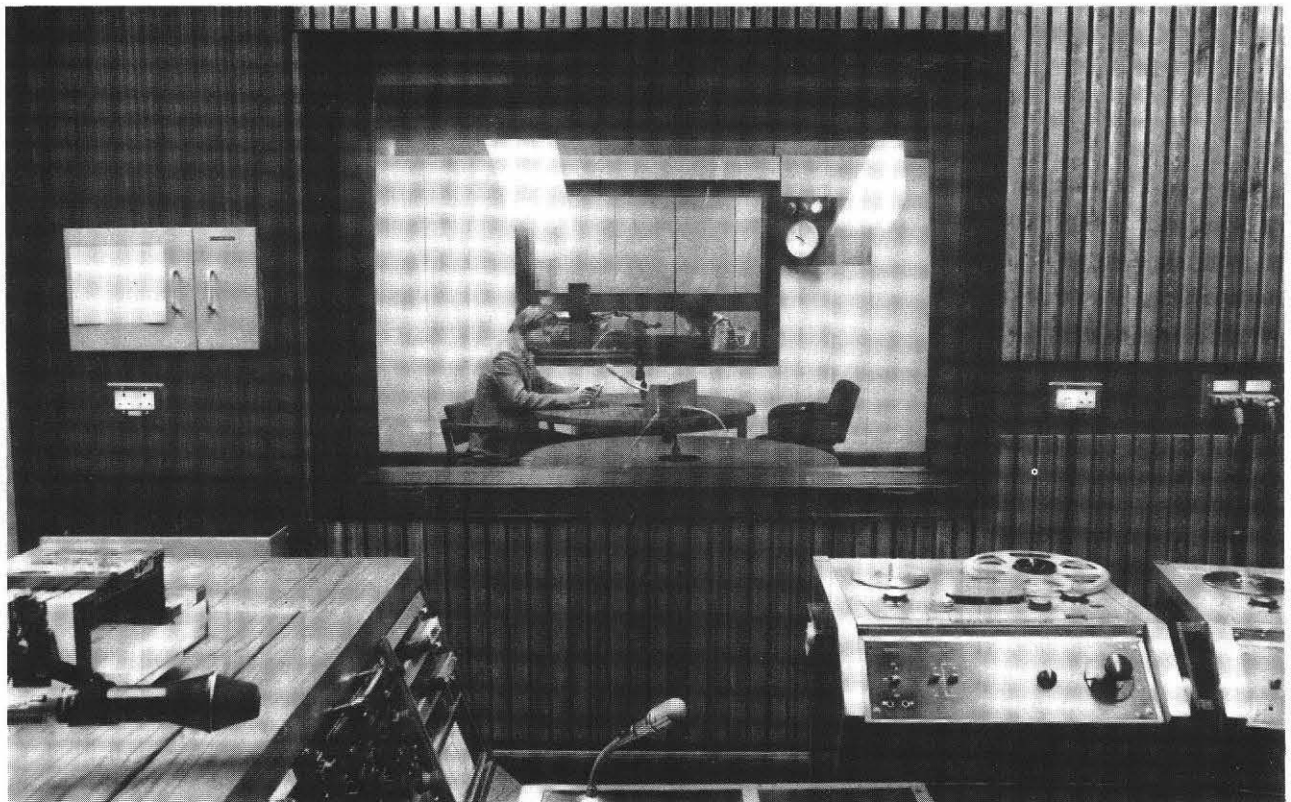
Fig. 8 Radio Manchester's Studio 1 with Cubicle 1B beyond, from Cubicle 1A. Each cubicle may be used alone or in conjunction with the studio, offering great flexibility for simultaneous rehearsal and transmission
