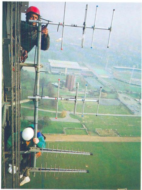
Experimental DAB antennae being installed on the Crystal Palace tower, as part of Eureka Project 147
