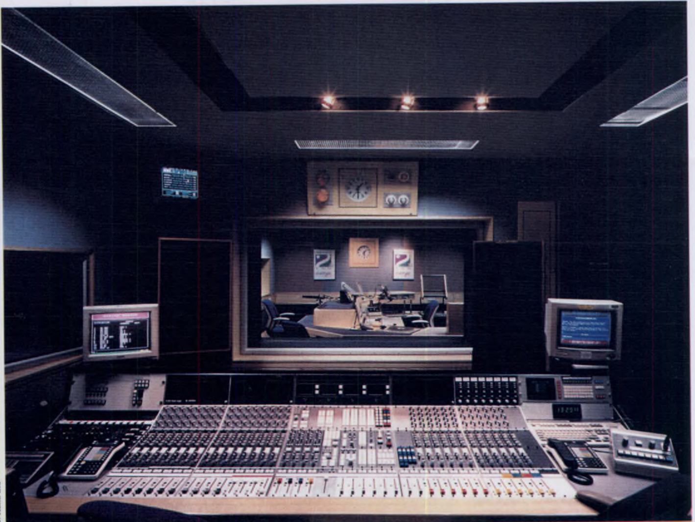
Suite 1G Cubicle with view of studio through the low-reflectivity window glass
