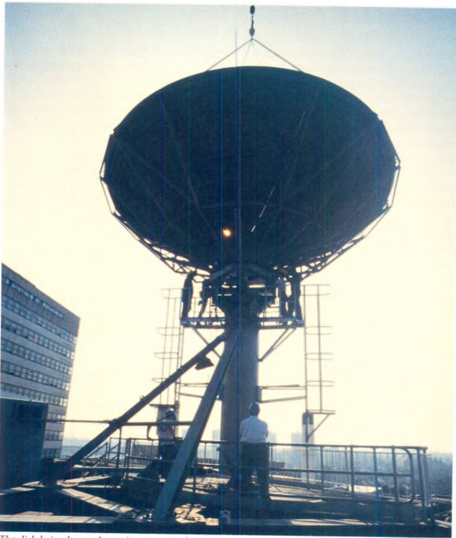
The dish being lowered onto its support column.
