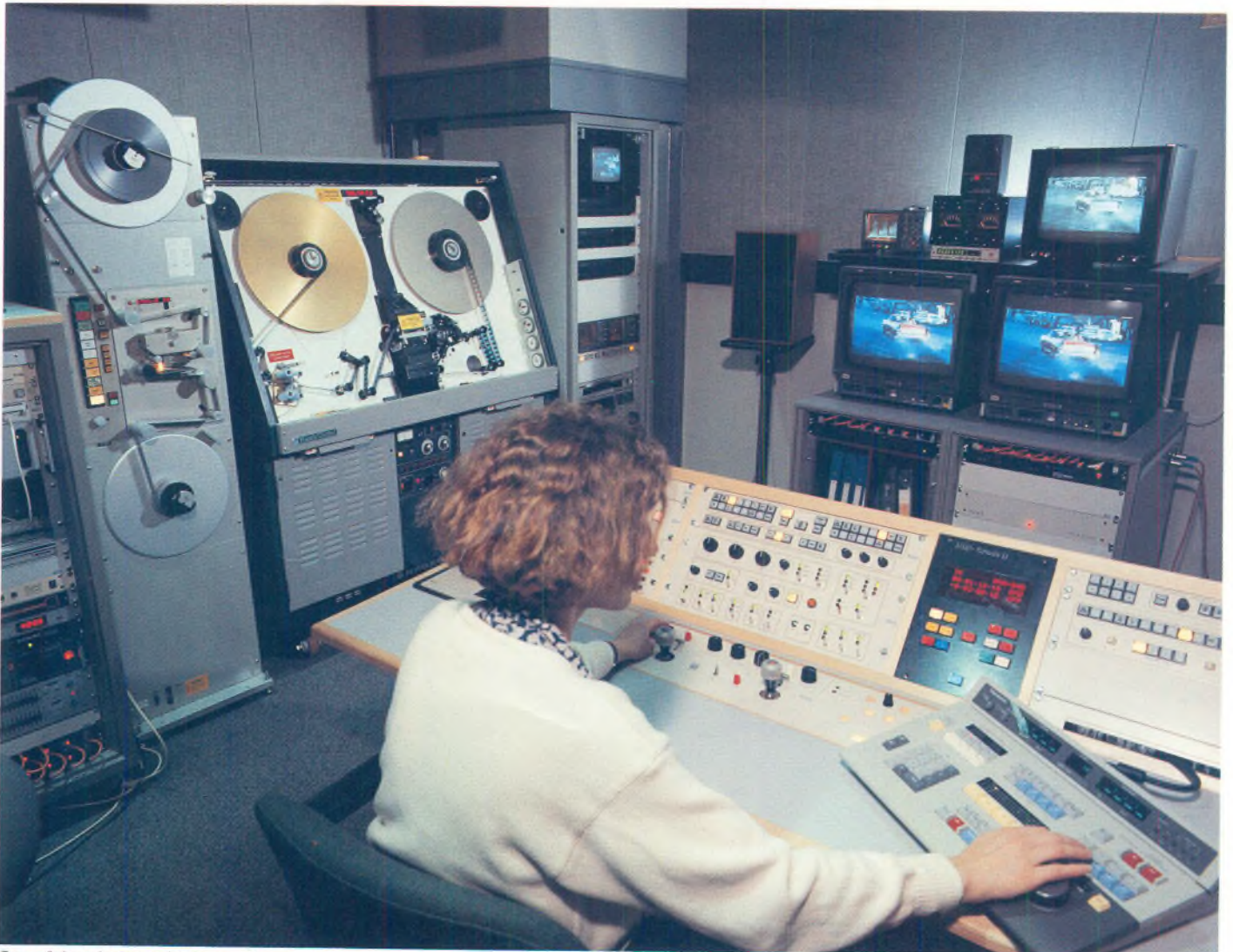
One of the telecine cubicles on Floor 1 (TK2).
