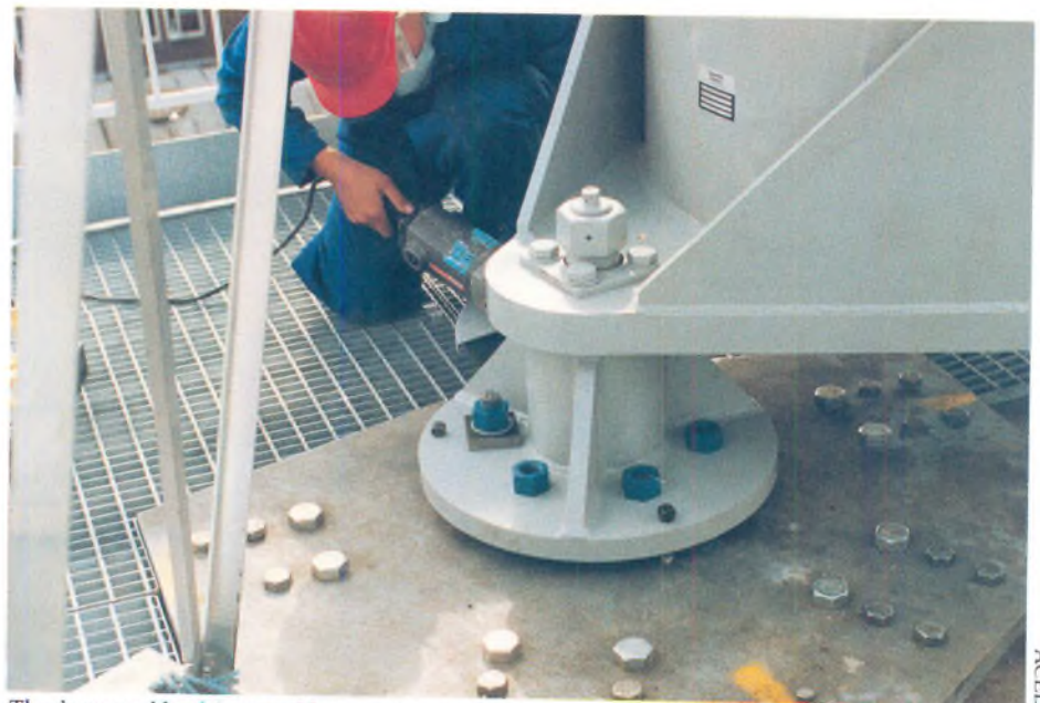
The downward load (approx 30 tonnes) is supported on a single bearing.
