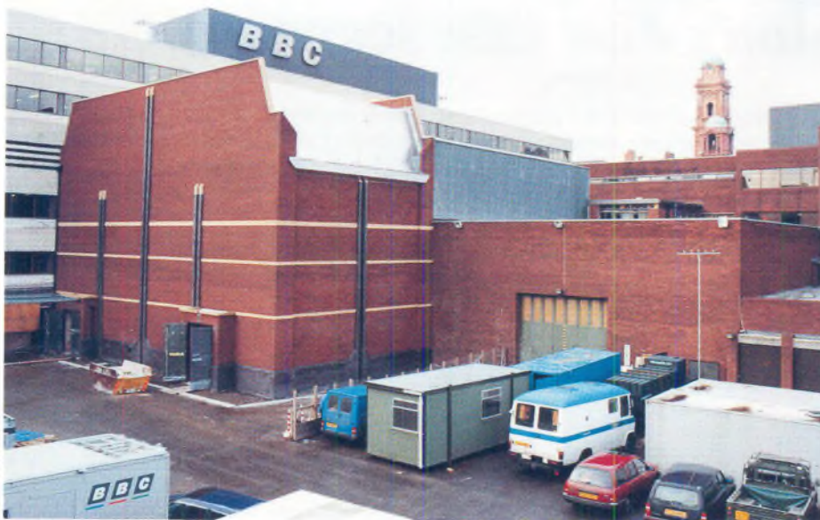
External view of the finished extension.
