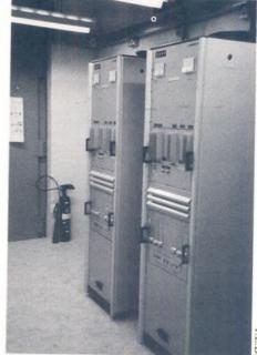
BBC1 and BBC2 solid-state transmitters at Newton (after re-engineering)
