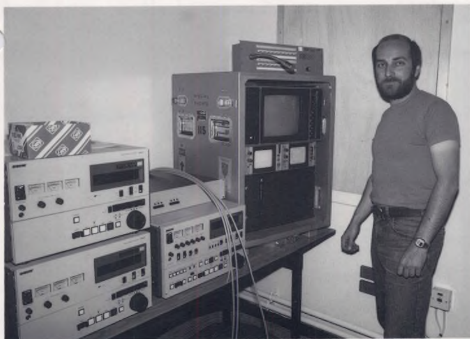
Canadian technician installer Graham Campbell alongside the Betacam half-inch VT machines arranged for editing. Note the equipment built inside the flight package.
