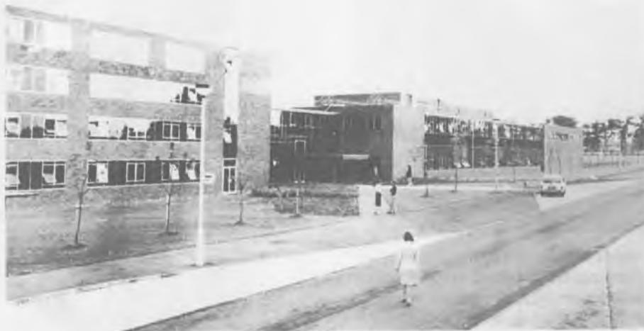
The Administration block, main entrance and reception. On the right, is the technical block.
