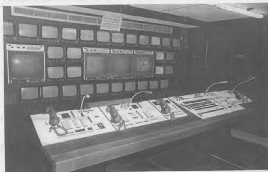
The rack of 34 monitors and the control desk in the extended production control room
