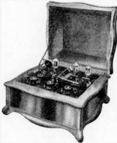
16. A Wireless Cabinet
