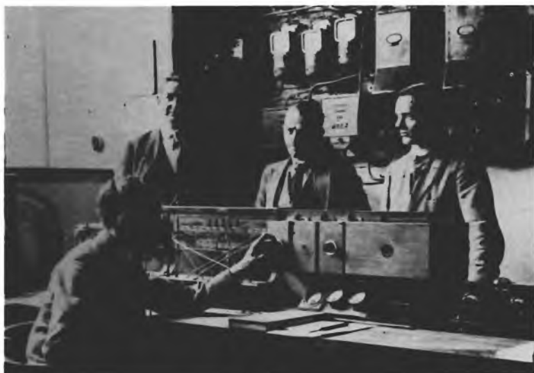
Control room, the Parsonage, Manchester, 1924
