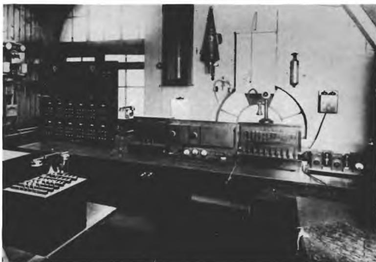
Control room, Aberdeen, 1929
