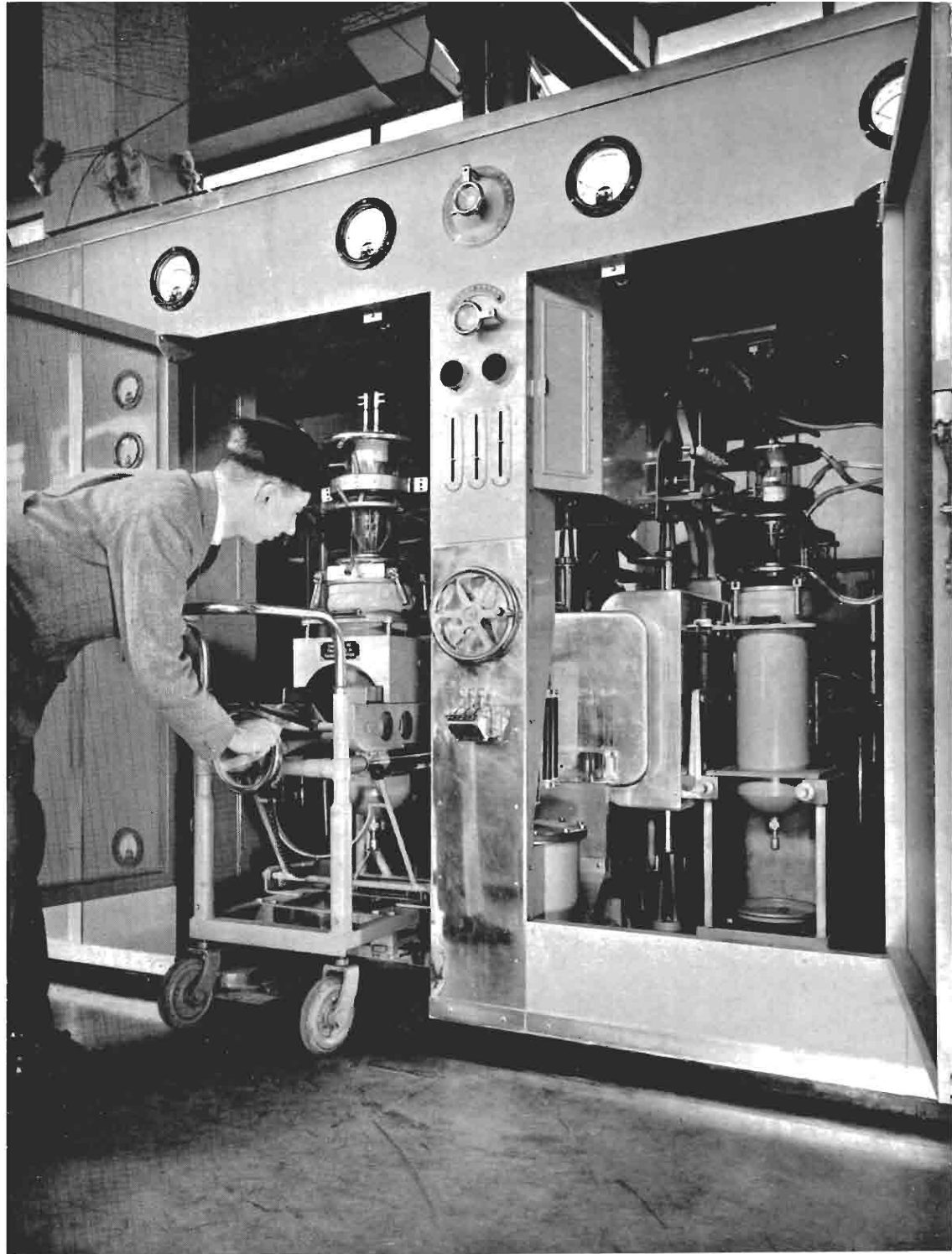
Large water-cooled valve being wheeled into position
