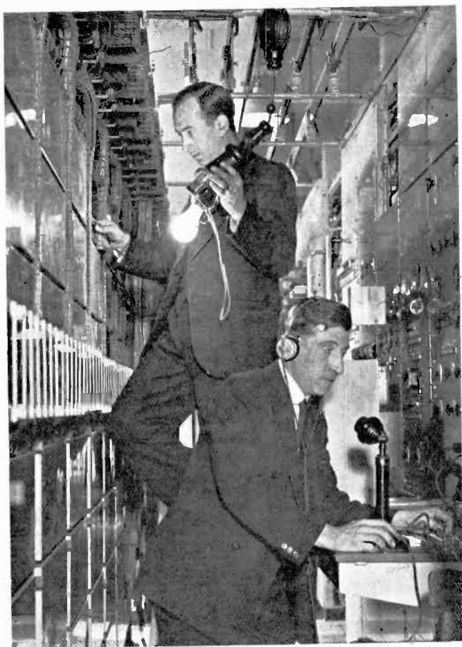
TESTING THE AMPLIFIERS AND LINES IN THE CONTROL ROOM
