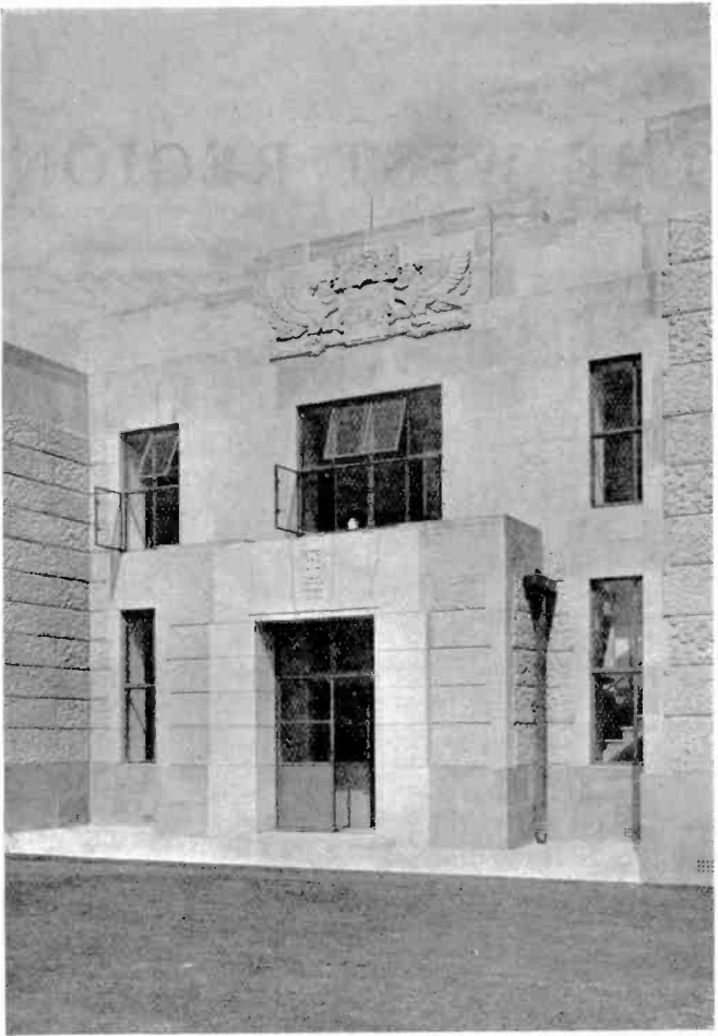
THE FRONT ENTRANCE TO THE WEST REGIONAL TRANSMITTING STATION
