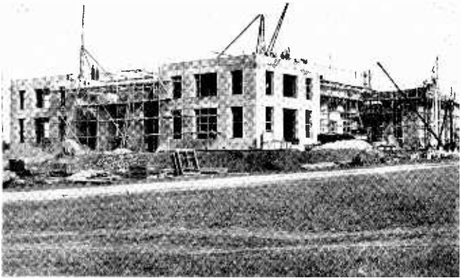
DROITWICH STATION UNDER CONSTRUCTION
