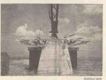
Foot of the aerial mast of the high-power broadcaster at Bisamberg (Vienna). Note the counterpoise wires anchored to the concrete base
