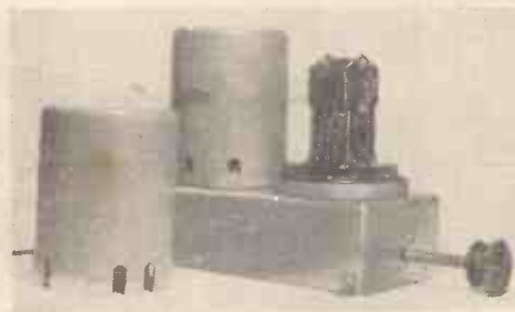
Another set of iron-core coils that can be used—made by Goltone
