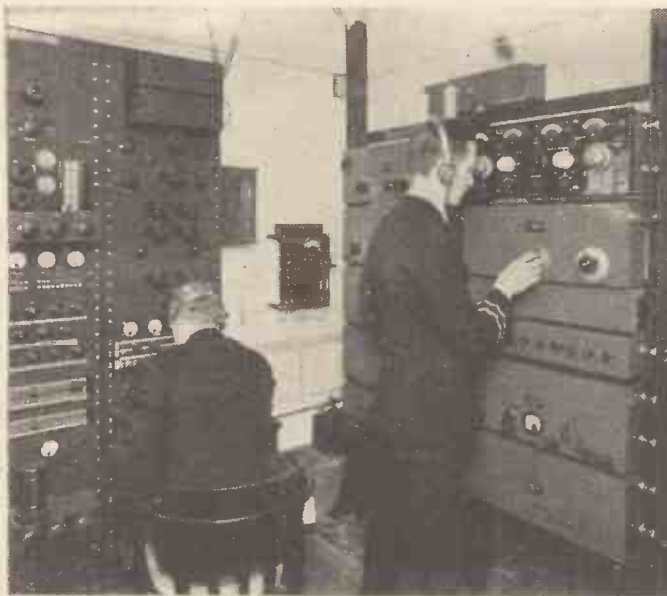
Marconi photo Telephone receiving-room on board s. s. Empress of Britain. The monitoring switchboard in front of the operator's chair enables the wireless-telephone equipment to be used from the ship's telephones
