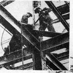
Radio marches on! Two striking views of the new Cossor factory now going up at Highbury. The height will be 75 ft. for the five storeys, for which 500 tons of British steel are needed. 60,000 sq. ft. of floor space will be available for over 1,000 workers.
