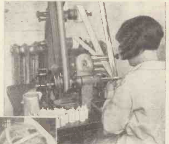
Winding and interleaving the paper and foil in the making of a typical T.C.C. condenser. The exact number of turns is noted on a revolution counter
