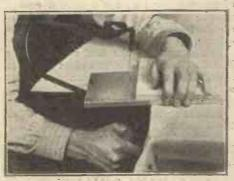
Thin sheet aluminium for screens or baseboards should be cut with a hacksaw between a "sandwich" of plywood or scrap wood so that a clean sawcut" edge results. Fretsaw holes in thin metal sheet should be cut in the same way with two pleces of scrap wood as a support, the hole being cut through metal and wood
