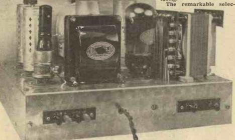
The basis of the receiver is a circuit consisting of variable-mu H.F. stage coupled by tuned-grid method to a screen grid detector which in turn is coupled to the power pentode output
