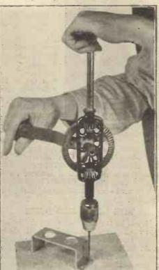
When drilling small holes in metal brackets and supports, keep the drill vertical and do not exert too much pressure on it. A nail can be put in the wooden board on which the metal piece is being drilled to prevent it turning under the drill
