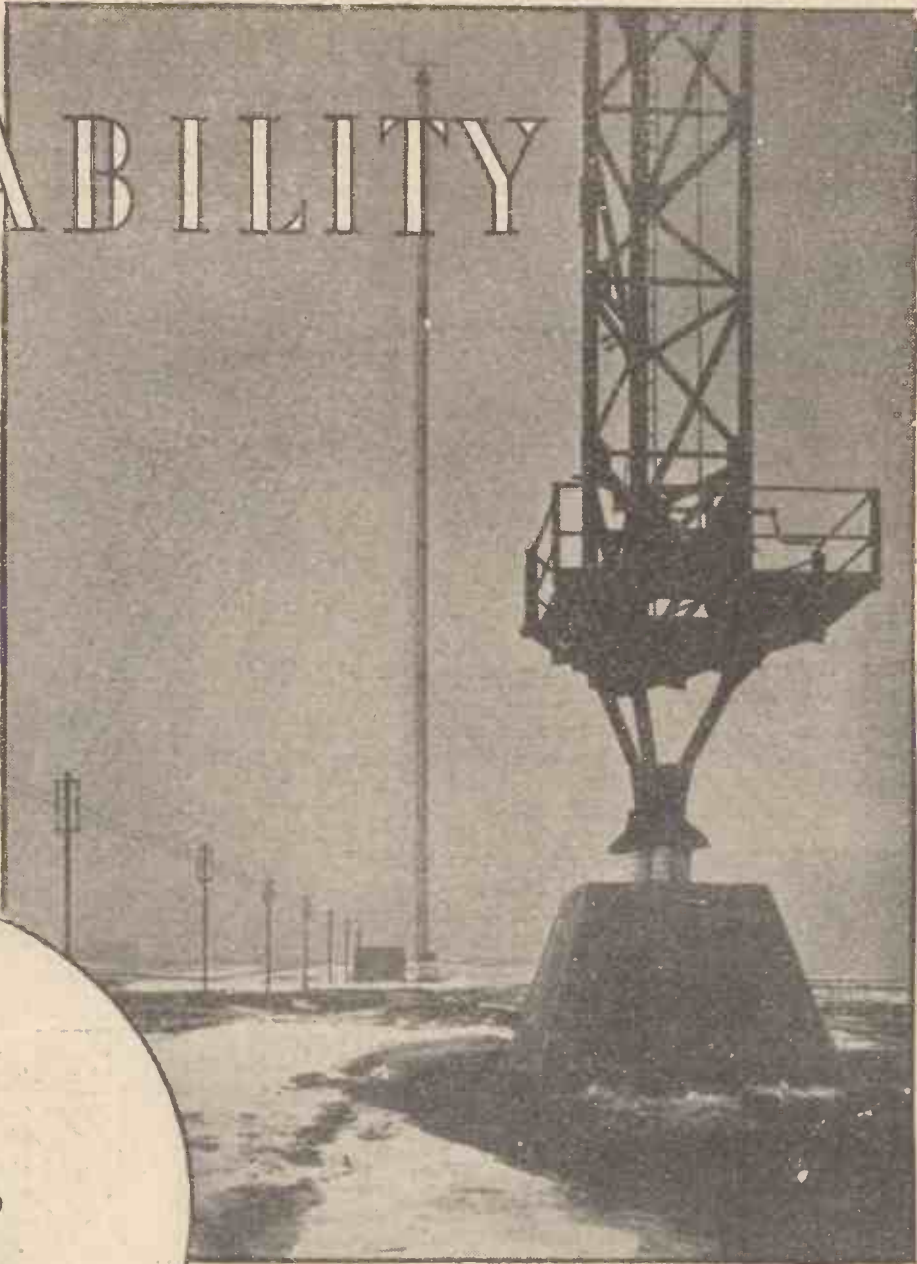
The Insulated Base of a 500ft. North Regional transmitter mast, with an aerial feeder but in the background.
