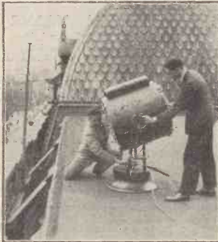
Fixing the searchlight speaker on the roof of the Marconiphone building, for the "broadcasting" of Big Ben
