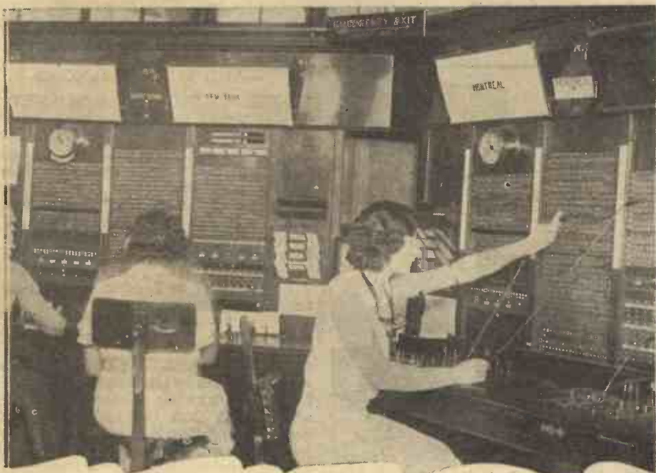
The heart of the Post Office radio system by which the B.B.C. now takes most of its transatlantic broadcasts and Canadian relays. These operators in London control the output through Rugby and handle the input from the Baldock super-het receivers
