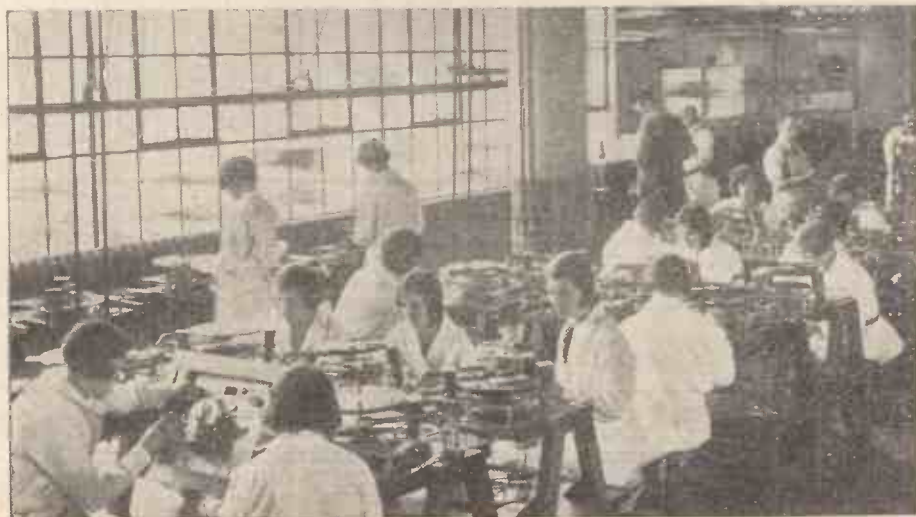
Special new plant has been installed in the H.M.V. factory for constructing the automatic record changing "robot" mechanism which is a feature of many of the new radio-gramophones. Note the overhead conveyors which carry the parts from one bench to the next.
