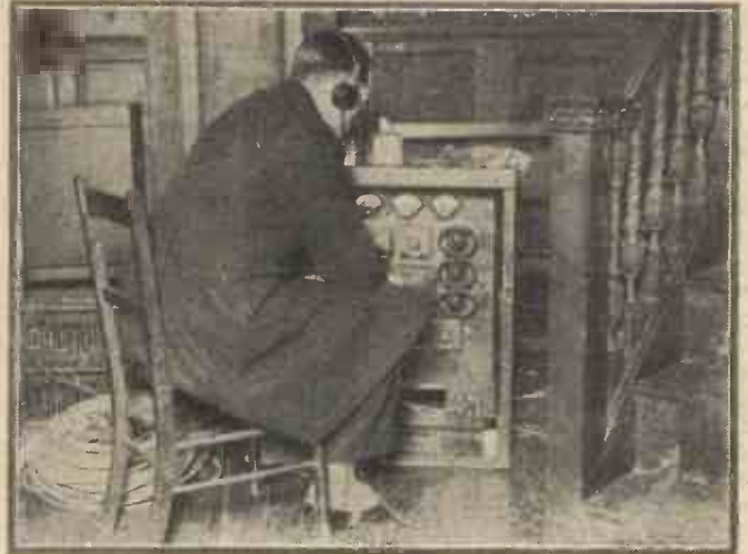
The portable amplifier in the basement at Downing Street
