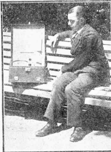
German portable sets are generally very compact, with ample metal screening. Here is a commercial portable in use.
