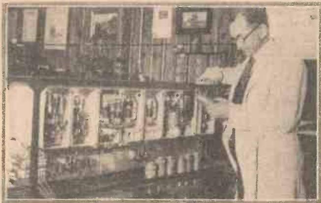
Testing the various units of the eleven-valve super-het used for re-broadcasting at Zehlendorf
